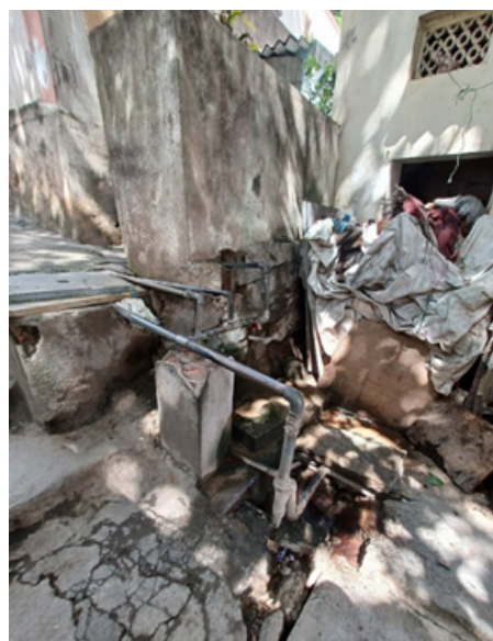
Pipelines are old and poorly maintained; often interchanged with sewage lines causing contamination
